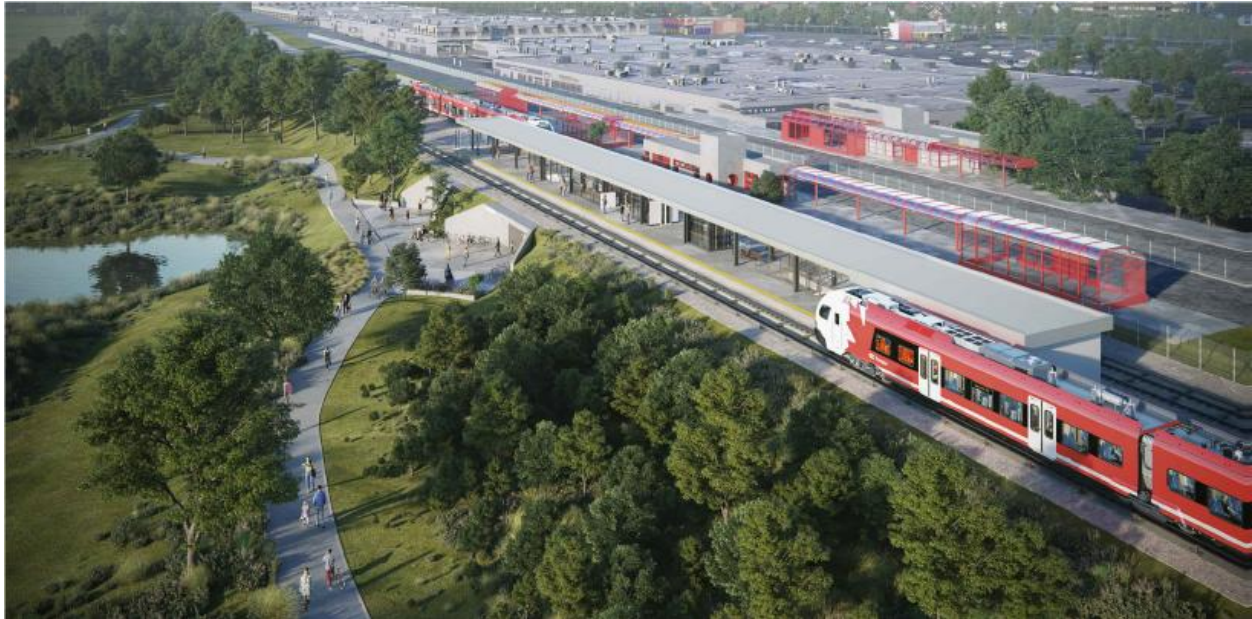
Figure 22: South Keys Station
