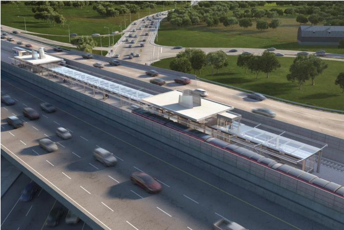
Figure 13: Montreal Road Station
