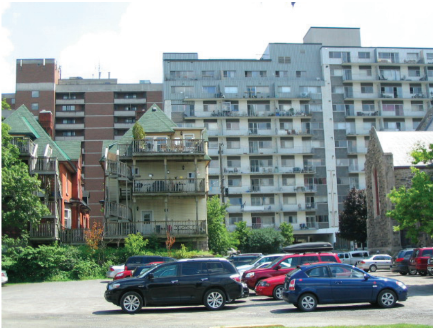
View south across existing parking lot showing portions of north elevations of Queen Street houses
