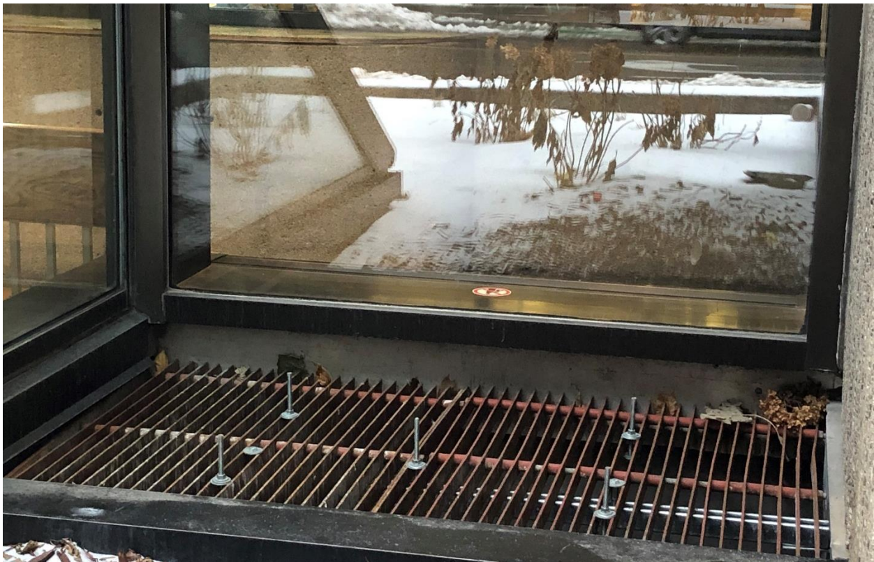
Figure 9: Open grate beneath reflective glass windows.
