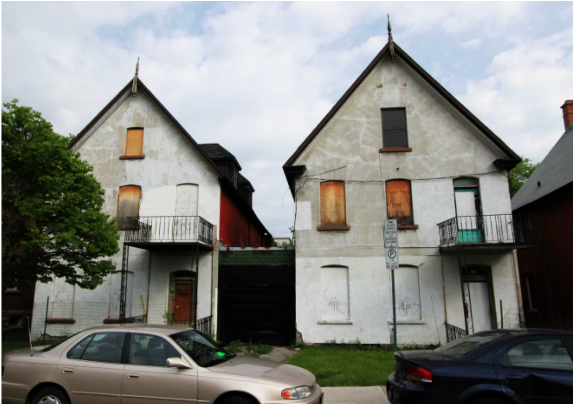
Figure 1. Wilbrod Street View
