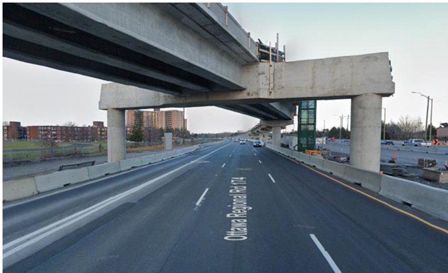
Figure 8: Straddle Bents
