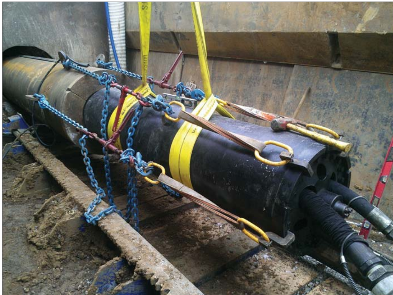
Figure 6: Pipe Ramming
