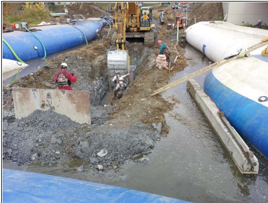
Figure 4: Open-Cut Construction using Cofferdams
