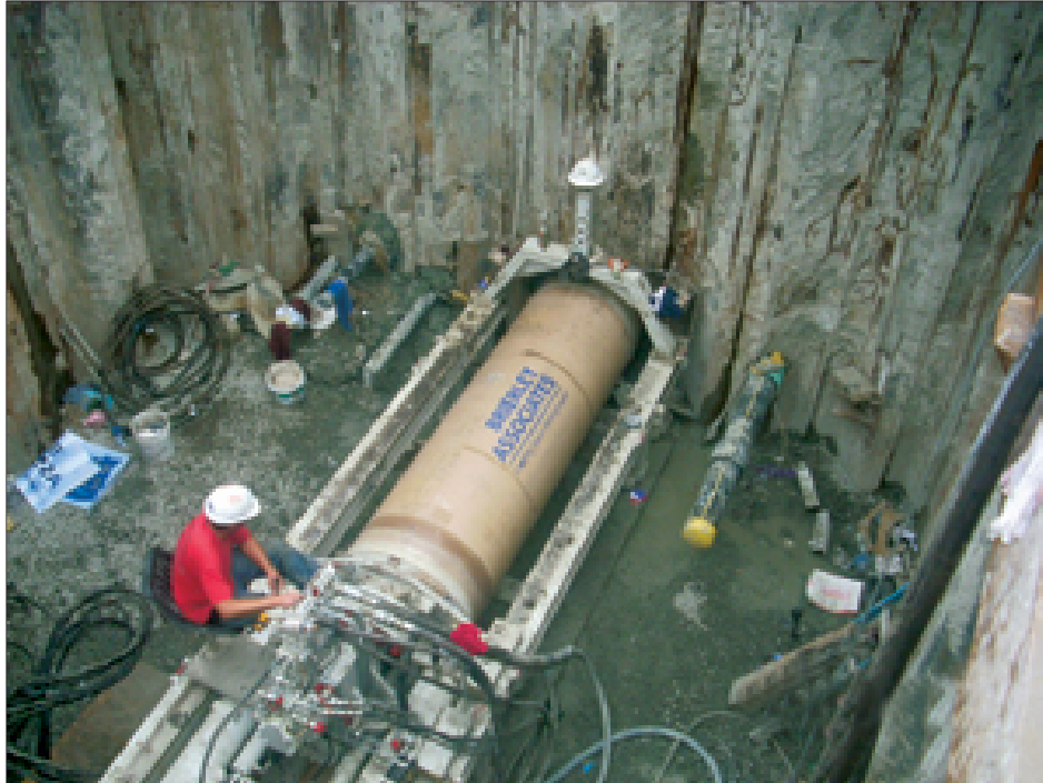
Figure 5: Auger Boring
