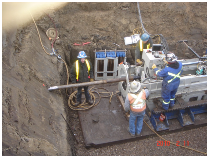
Figure 10: Horizontal Rock Bore
