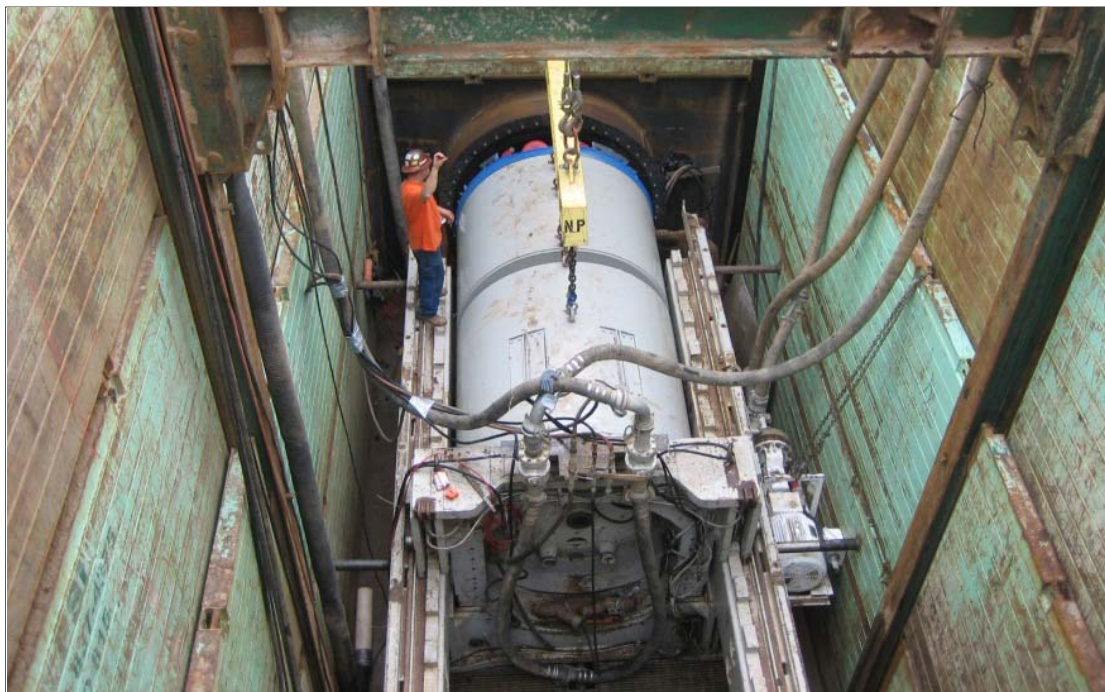
Figure 7: Micro-tunnelling
