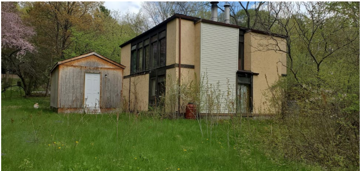
Rear façade of 8 Briarcliffe Drive with existing detached garage (left).
