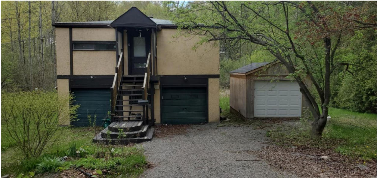
Front façade of 8 Briarcliffe Drive with existing detached garage (right).
