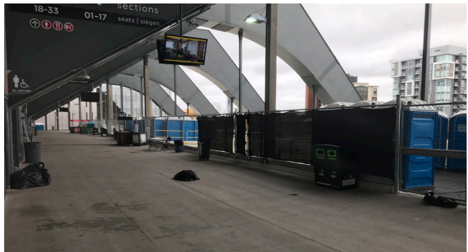
Temporary toilet facilities permanently used
