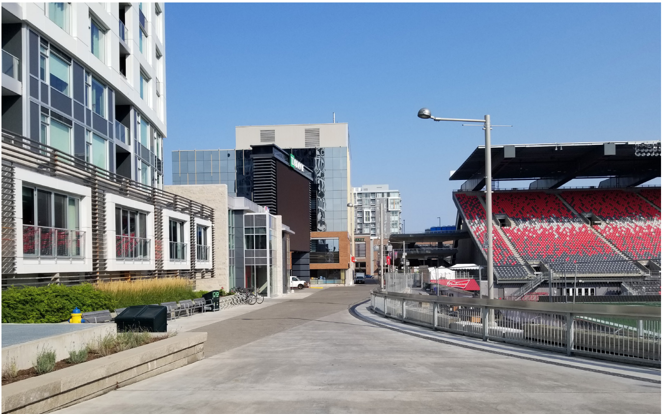
North Grandstand context
