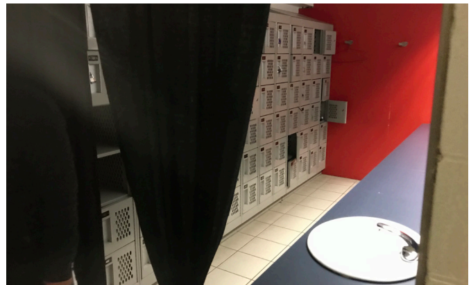
Washroom converted to locker space
