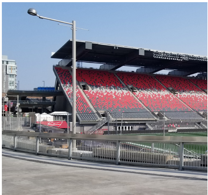
TD Place Stadium North Grandstand
