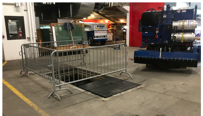
Ice melt pit obstructing circulation/marshalling space
