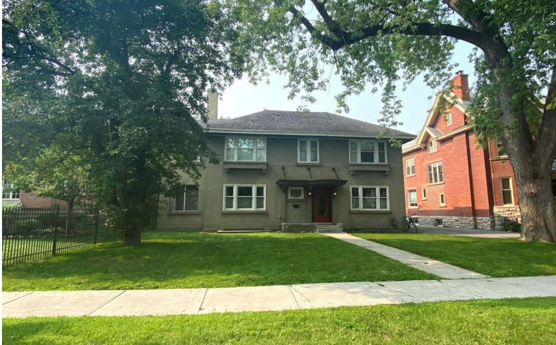
View of existing two storey house from the street.
