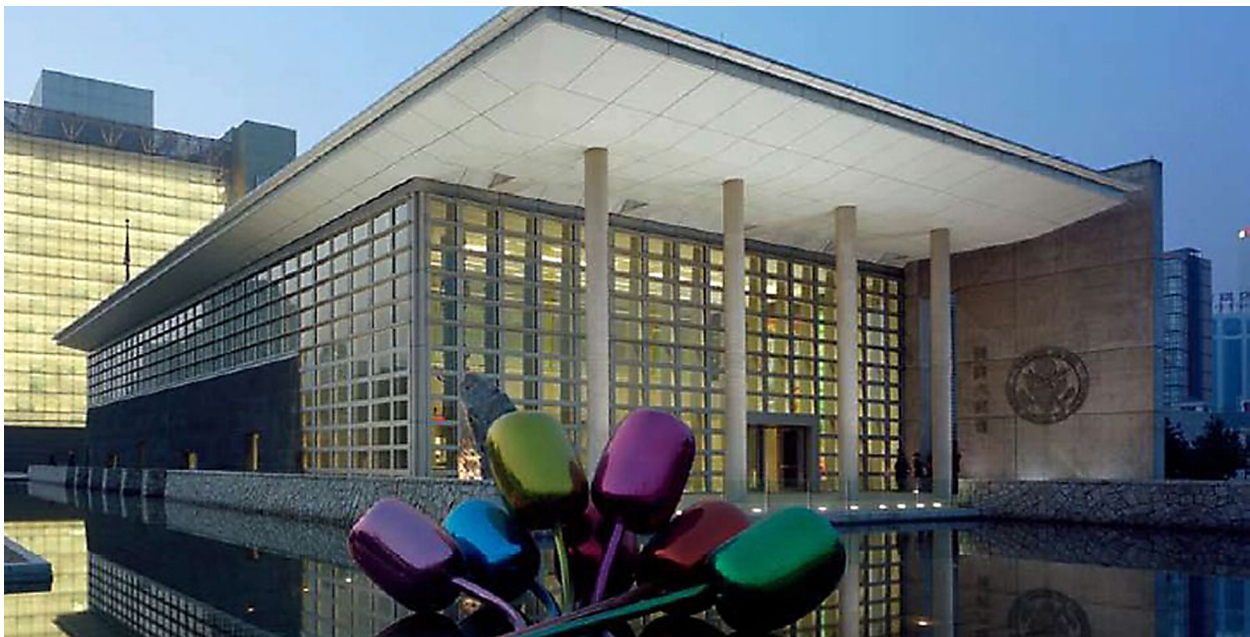
Integration of security with the landscaping and the siting: a reimagined moat, USA Embassy in Beijing. Architects : SOM; landscape architecture : PWPLA, Source : http://www.pwpla.com/
