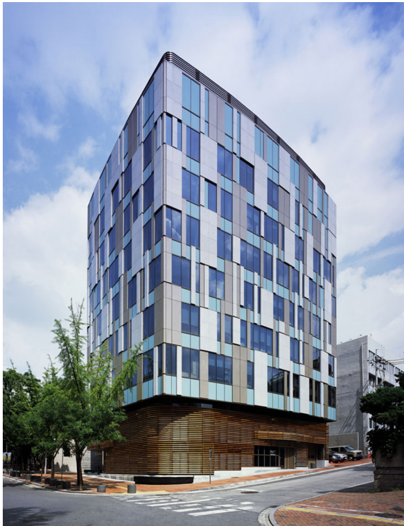
Contemporary architectural expression, Canada Embassy in Seoul. Architects, Zeidler Partnership. Source : http://www.zeidler.com/
