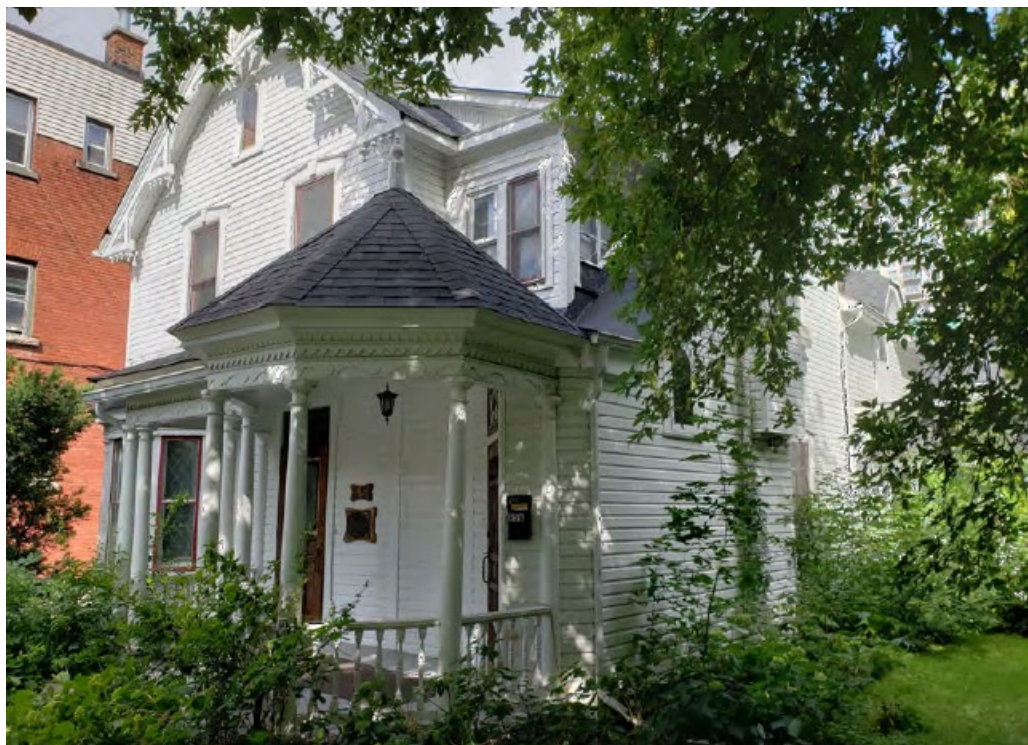
Front Elevation (from southeast)
