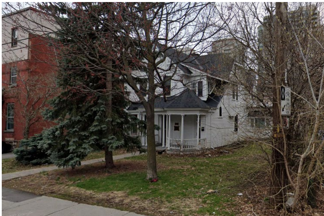
Front Elevation (from southeast)
