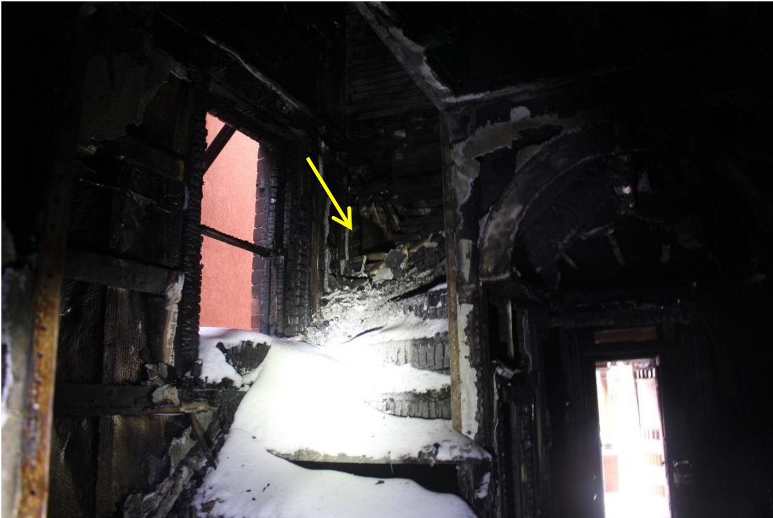
Photograph 8: View of second-storey stair structure.
