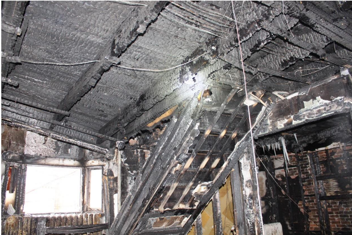
Photograph 4: View of the second-storey floor framing.
