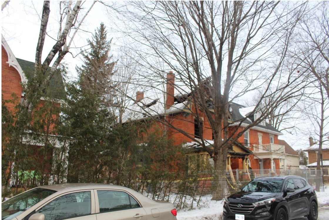
Photograph 2: Partial view of the west side elevation of same.
