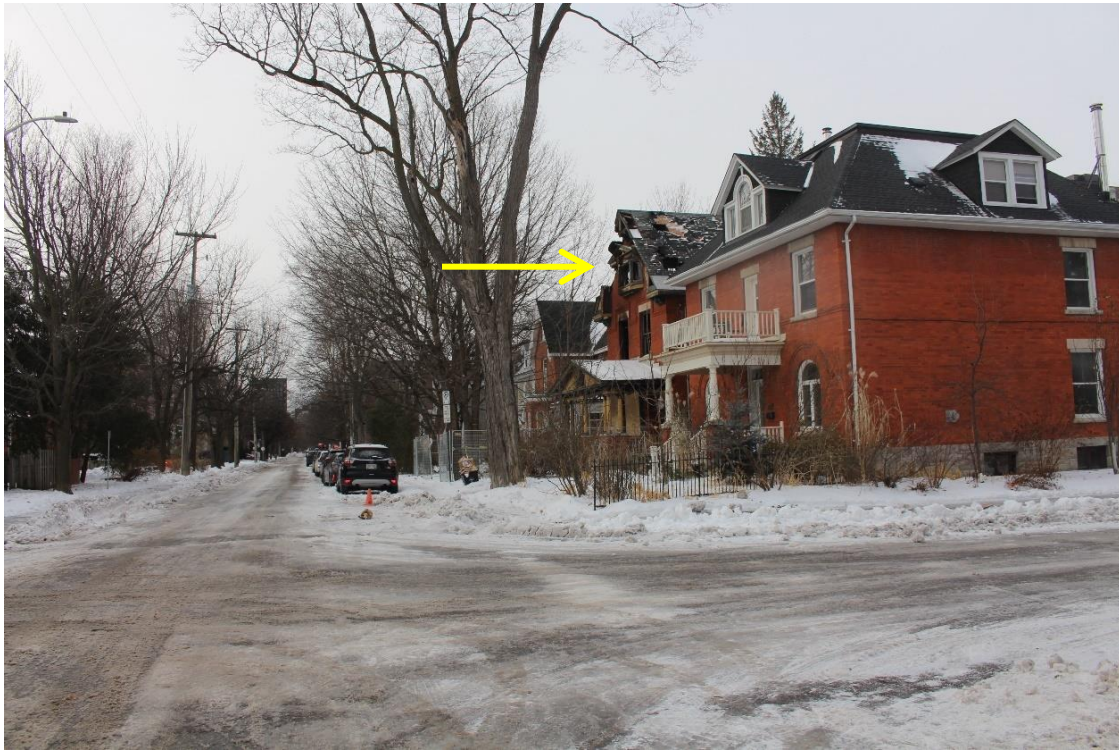
Photograph 3: Partial view of the east elevation of same.
