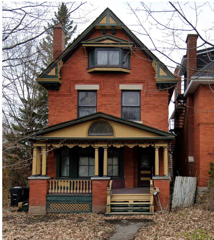
Figure 1: 323 Daly Ave. prior to fire [Google maps, 2019]
