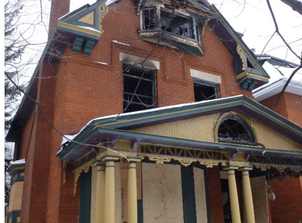
Figure 3: Brick masonry, south façade [JCAL 2021]
