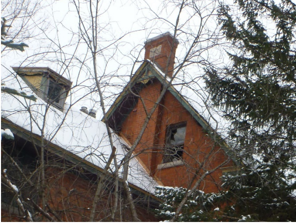
Figure 6: North chimney in good condition [JCAL 2021]
