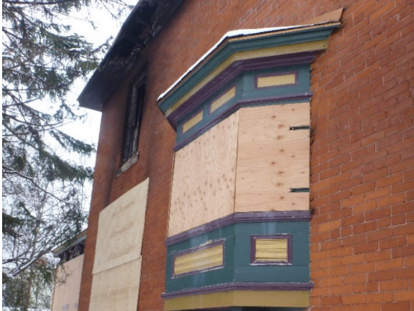
Figure 2: Brick masonry, west facade [JCAL 2021]
