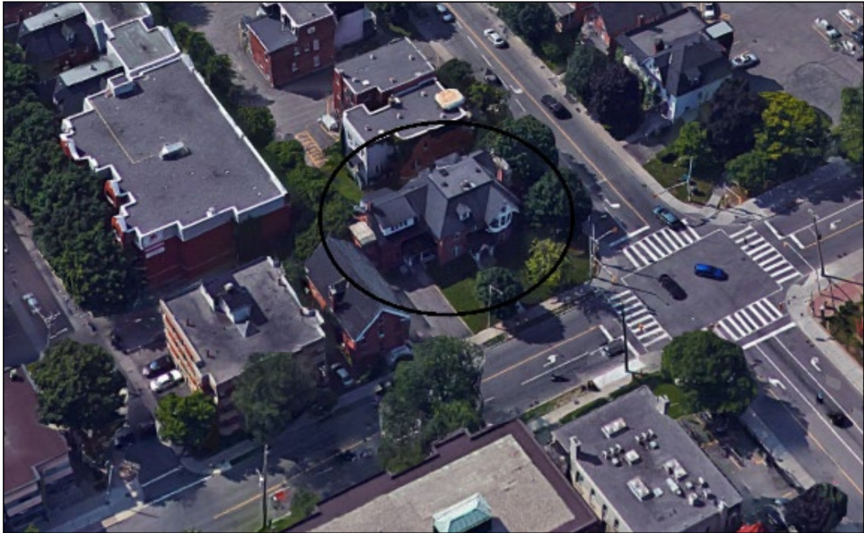
Aerial view of 190 Laurier Avenue East (circled) on the corner of Laurier Avenue and King Edward Avenue showing surrounding properties (Source: Google Earth).
