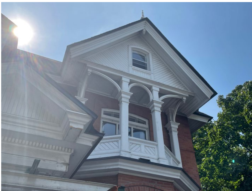
Second storey balcony with decorative wooden elements.
