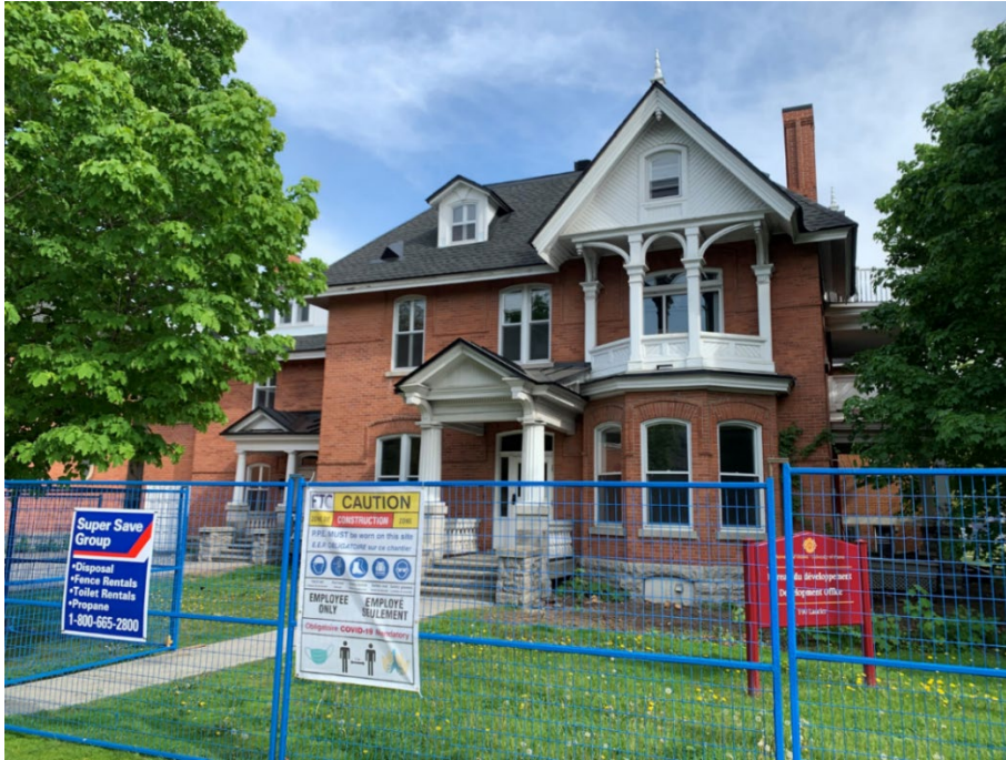
Front elevation of 190 Laurier Avenue East.
