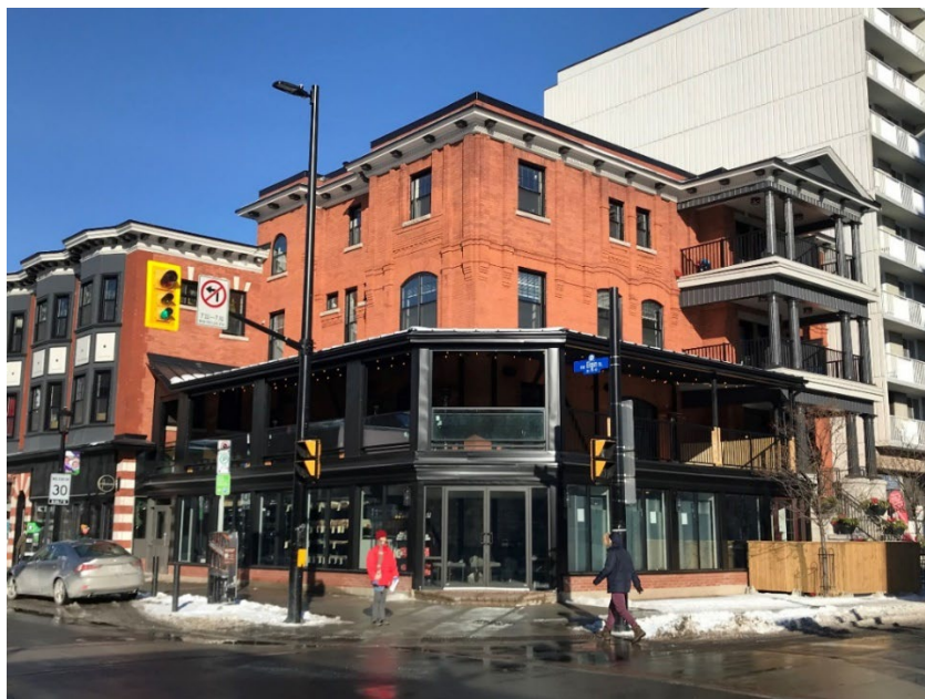
View from southwest corner, December 2021
