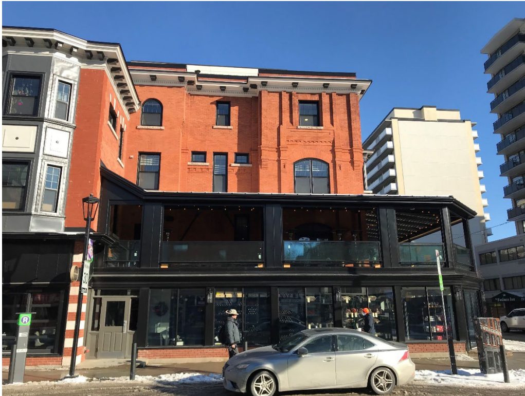
View of Elgin Street façade, December 2021
