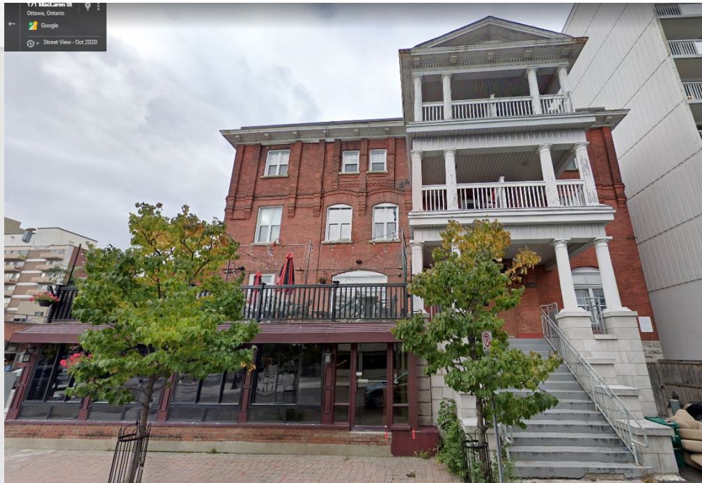
View of MacLaren Street façade, Google Streetview 2020
