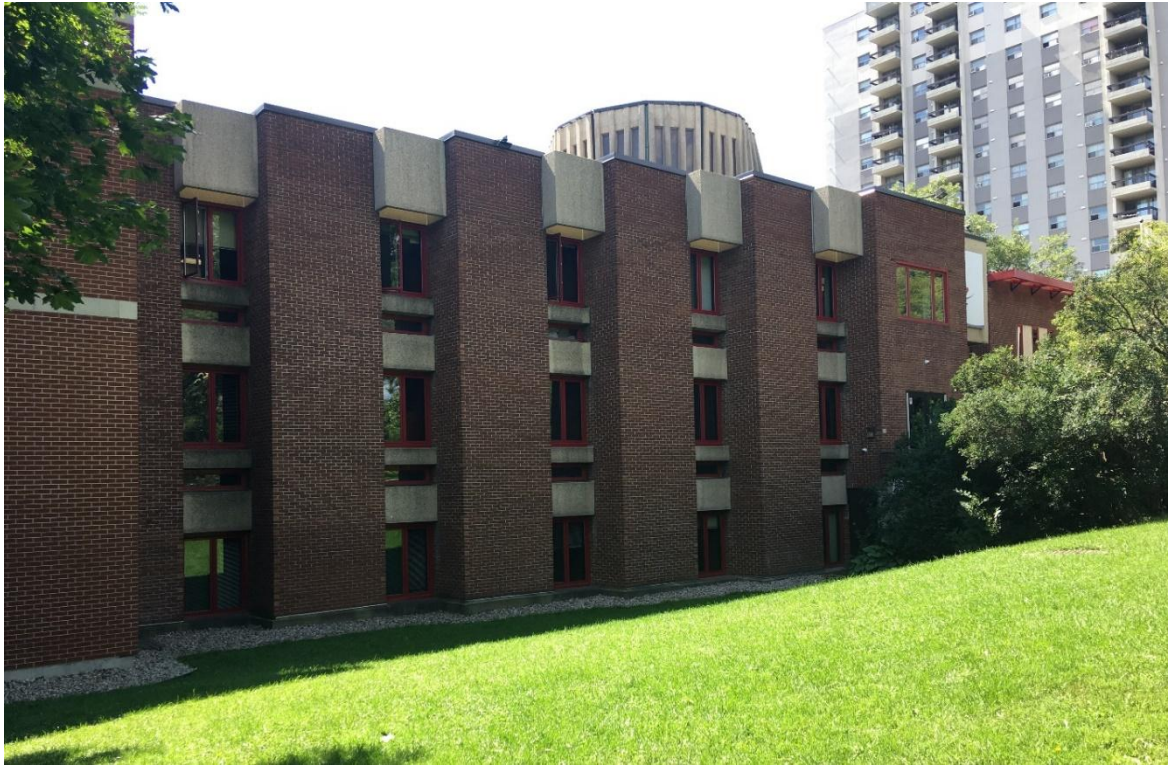
View of the east façade, from the south.
