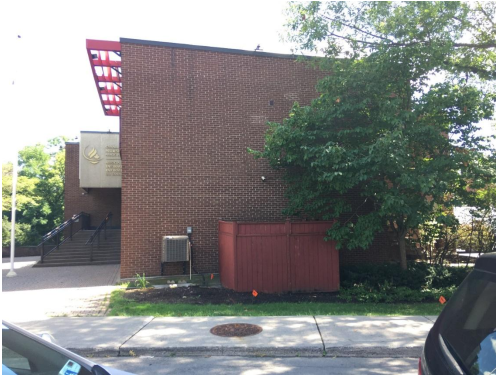
View of the north elevation from Lewis Street.
