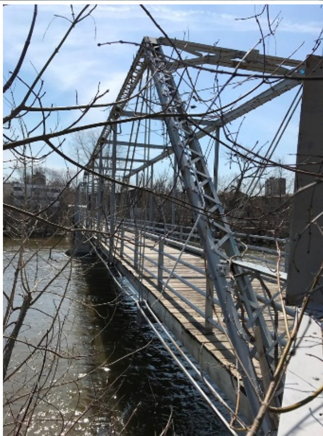
Top Left: View of Porter's Island Bridge looking east. Source: © Google 2019.
