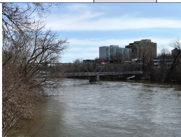
View of Porter’s Island Bridge looking east, 2017. Source: City of Ottawa.
