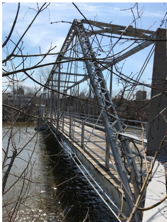
Porter's Island Bridge, view looking along bridge, 2018. Source: City of Ottawa
